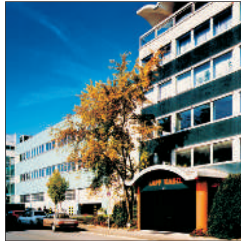
The Lapp Kabel headquarter in Stuttgart-Vaihingen.
